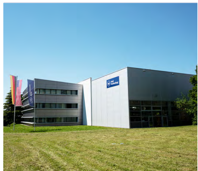
Weil Technology, plant 2 Müllheim
