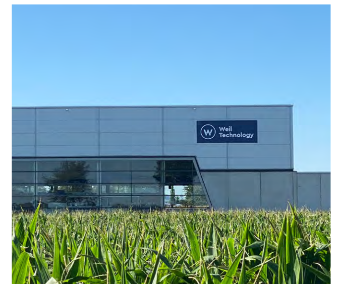
Weil Technology, plant 2 Müllheim
